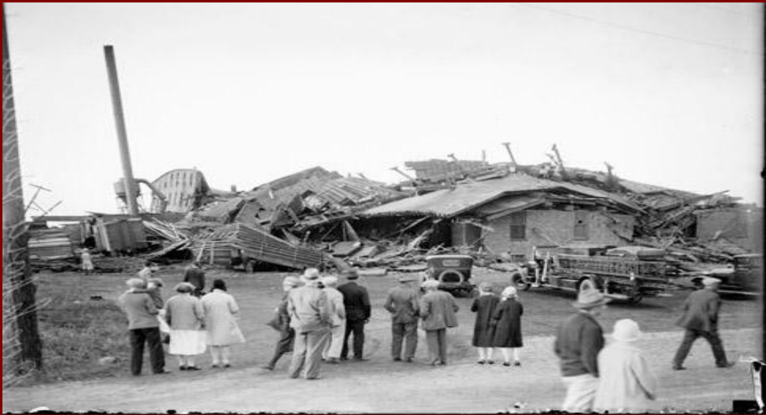
Spectators standing on a dirt road, looking at a house damaged by a tornado. Illinois 1928. Photographs from the Chicago Daily News, 1902-1933 American Memory, Library of Congress
